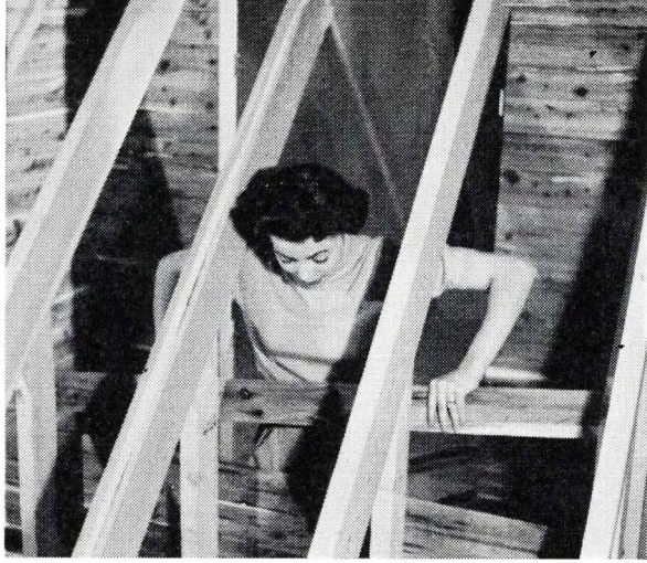
Fragrant do-it-yourself cedar boards are tongued-and-grooved on all sides for quick and easy construction.
